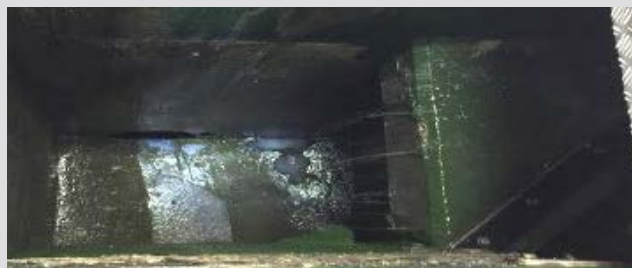
Figure 3.1 Damaged coating
