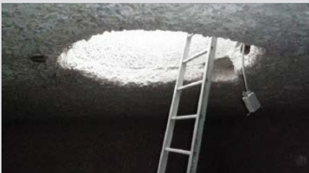
Figure 2.1 Wet well high-pressure cleaned and abrasive sweep sandblasted
