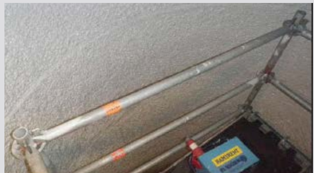
Figure 2.2 Surface of wet well with final coat of protective coating for concrete
