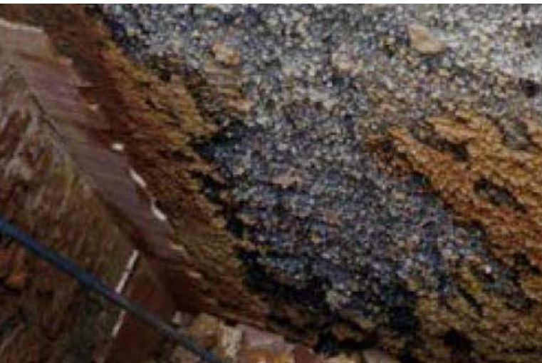
Figure 2. Biogenic corrosion in enclosed head space of concrete bar screen chamber
