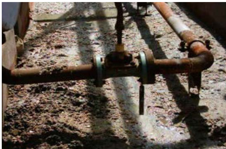
Figure 3. Acid attack of concrete in sulfuric acid containment
