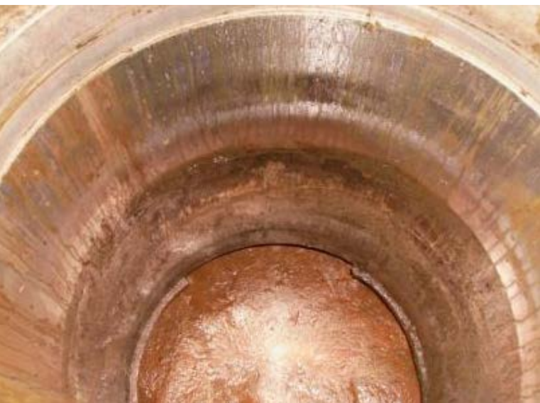
Severely scratched barrel as a result of metal-to-metal contact with the ram
